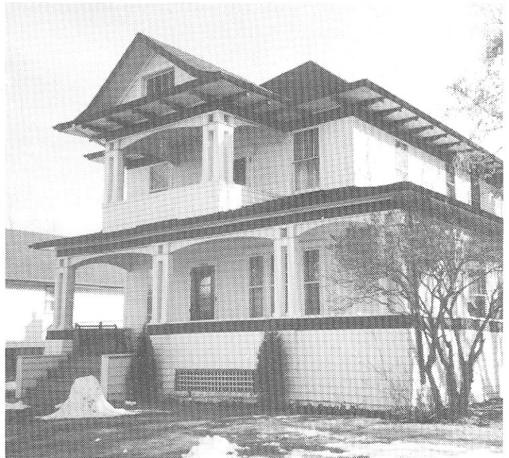
The Chown residence has a semi-tragic history, reflecting the boom-bust economic cycles of Edmonton.
